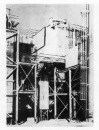
**BUELL PRECIPITATOR** with vertical inlet duct. Horizontal baffle pipes have been installed in duct to improve gas distribution and increase efficiency. Frame on which baffles are mounted extends downward at about 20° angle.
